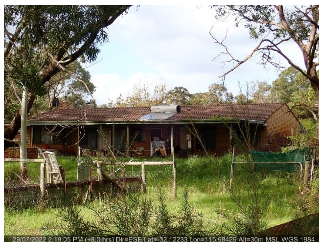
Photo ID: Photo 8 Looking at the neighbouring dwelling. Note the photograph was taken outside of the firebreak notice applicable period.
